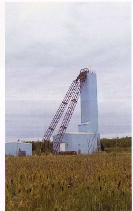
The Taylor Project headframe at the Stock Gold Complex.
