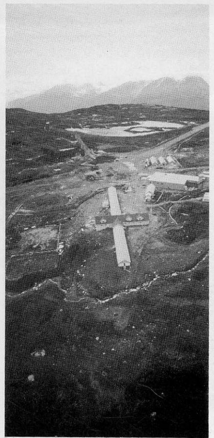
The Johnny Mountain mine, north-western B.C.
