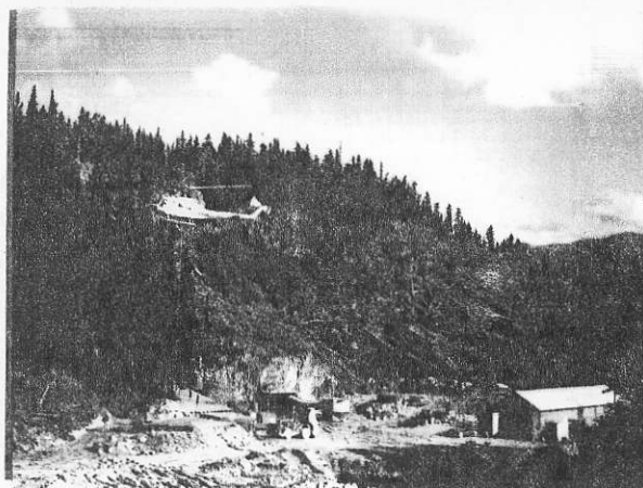
Figure 5 THE BELL-205 HELICOPTER IS DELIVERING A LOAD OF 350 GALLONS OF FUEL. THE PORTAL OF THE EXPLORATION DECLINE IS IN THE BACKGROUND.
