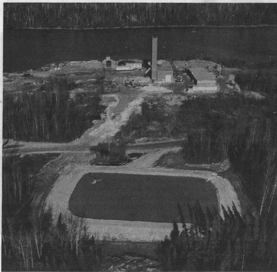
A view of the Norlartic minesite area near Val d'Or, Quebec, where Aur Resources is currently completing an underground program.
