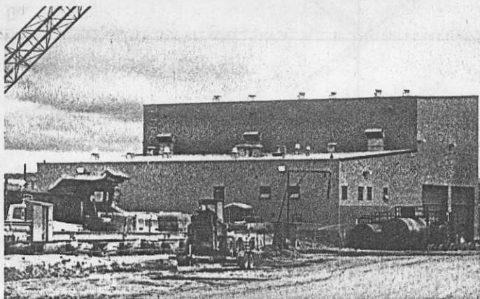
The new pit shop with service vehicles in the foreground
