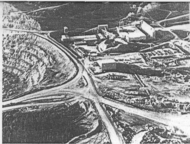
The Endako plant sits beside the 355-acre open pit (Placer Development Ltd photo)
