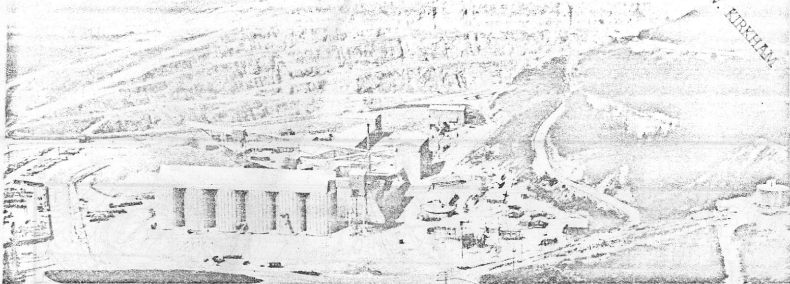
Endako: Overlooking the mill area
