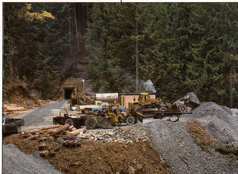
Upper adit, September 1987
