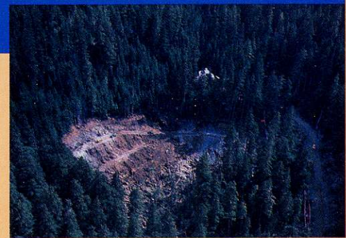
TUNNEL PORTAL SITE PREPARATION.
