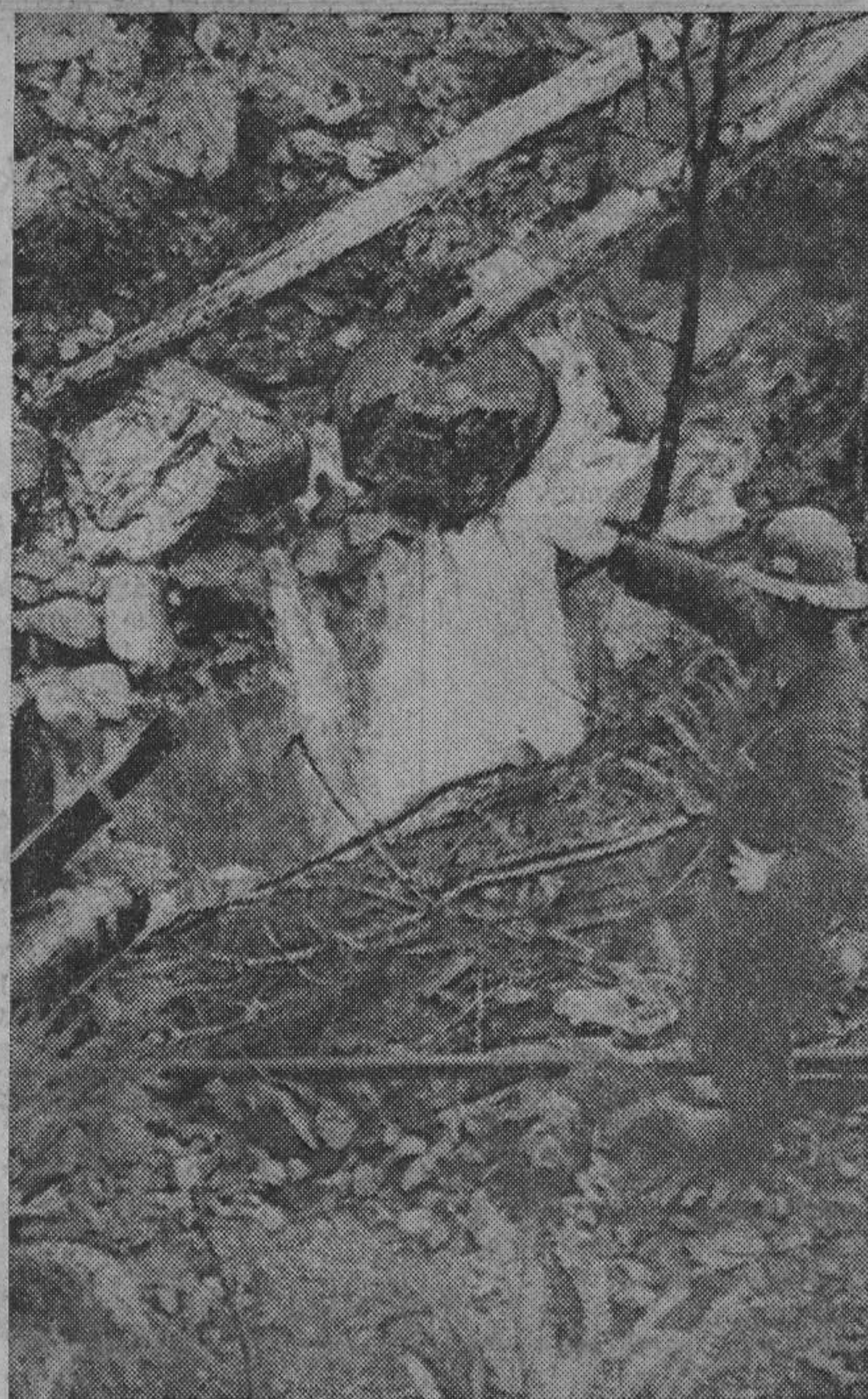
HOLE IN RIVER BED of Jordan River sucks in water and dumps it down 300 feet into copper mine. Gravel will be dumped into the hole to plug it, and concrete cap will seal off the cave-in.
