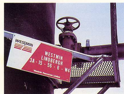
Site of Westmin's first enhanced recovery pilot project
