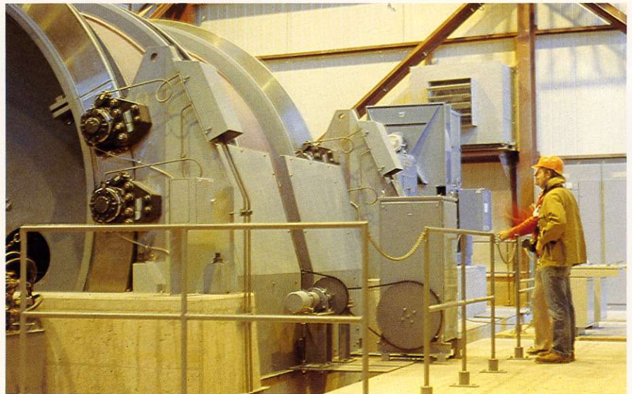
The main hoist for the new H-W shaft
