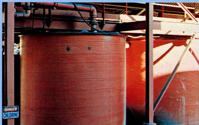
Unique alkaline chlorine plant at mine concentrator installed to ensure high environmental standards are maintained.
