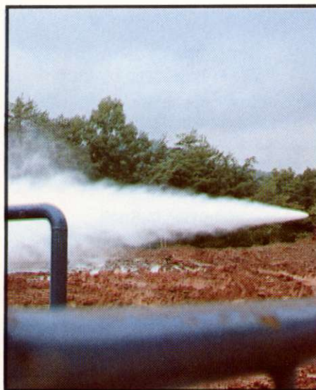
Blowing off the frac fluids at a well in Grandview Township, Ohio.
