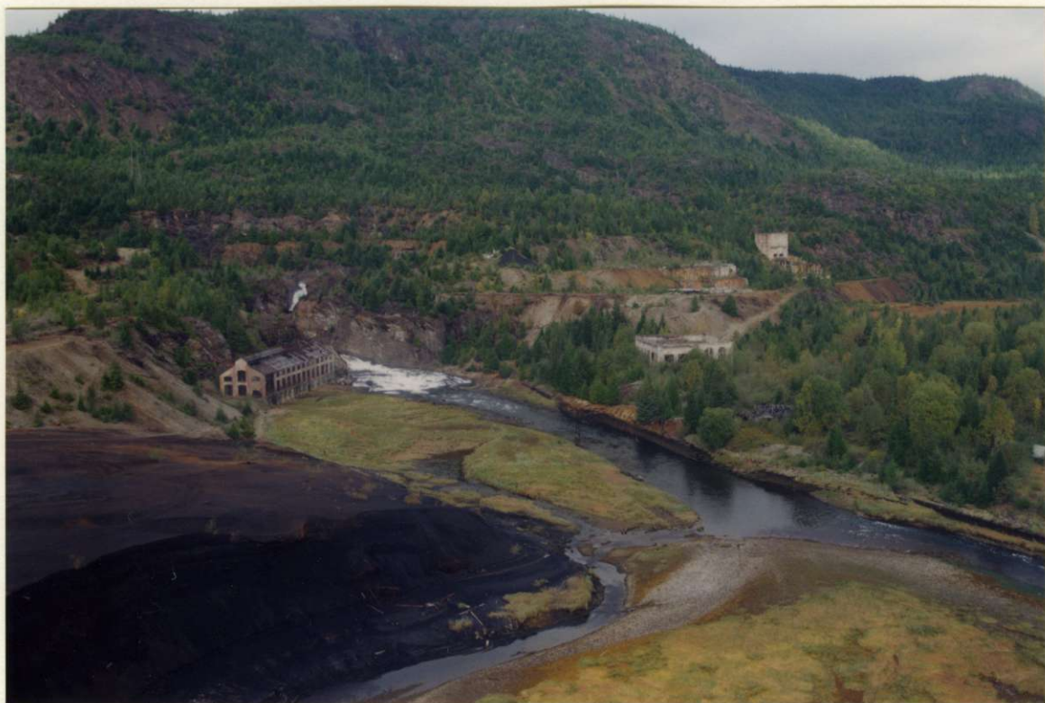
ANYOX TOWNSITE AT THE MOUTH OF ANYOX CREEK. BLACK TAILINGS LOWER LEFT CONSIST OF 85-95% SILICA WHICH IS RECLAIMED FOR ABRASIVES.
