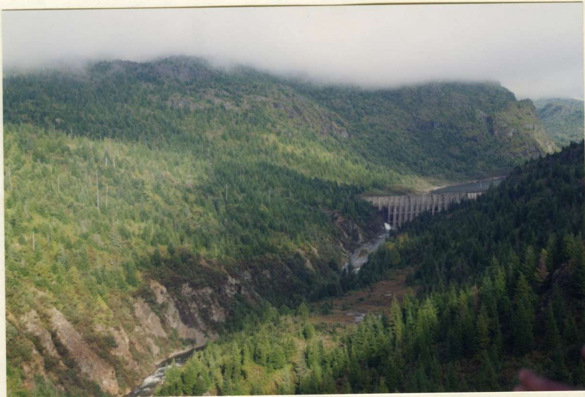
ANYOX CREEK HYDRO DAM LOOKING NORTH.
