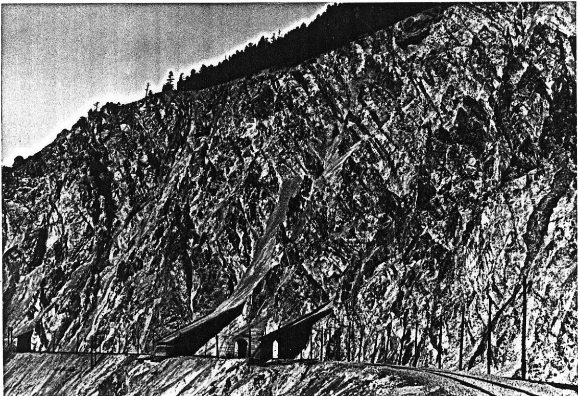
B. Close-up view of A; compare position of rock sheds. Bleached foliated leucocratic intrusive with discontinuous limonite-stained mafic dykes and sills.
