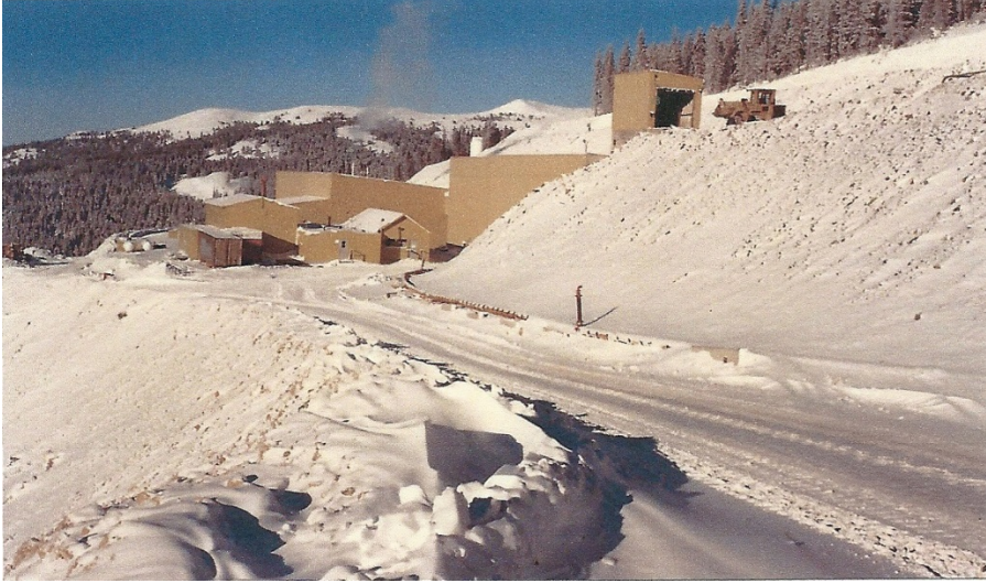
The Blackdome mill, shop, lab and power-house complex
