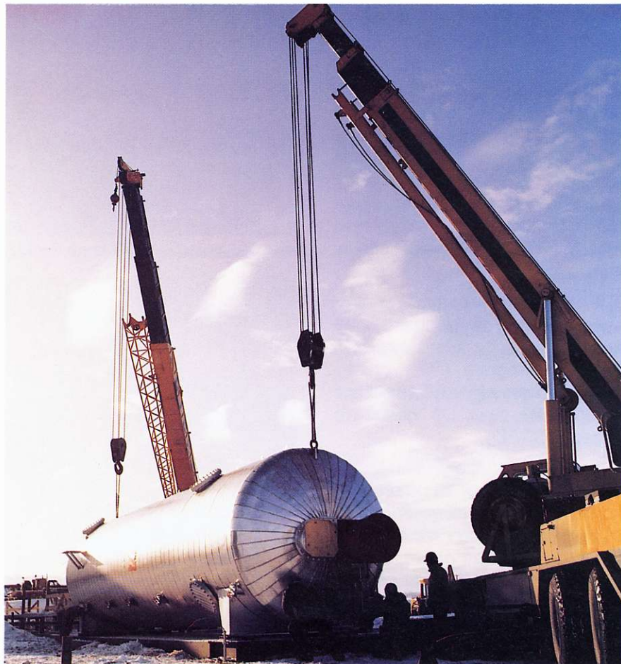
A massive vessel being lifted into place as part of the new cleaning plant which came on stream late in the first quarter of 1984.
