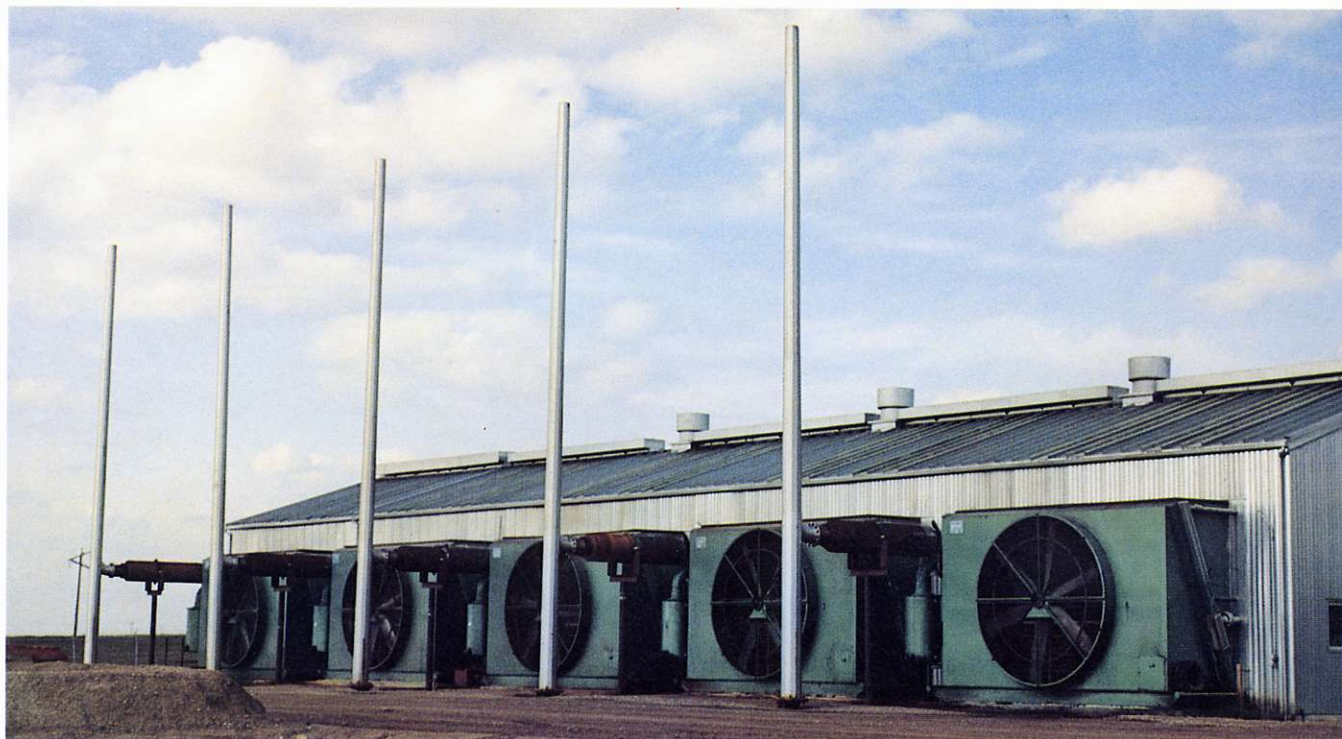
Rear view of one of Westmin's gas plants showing series of fans used to cool the compressors and the natural gas being pumped.
