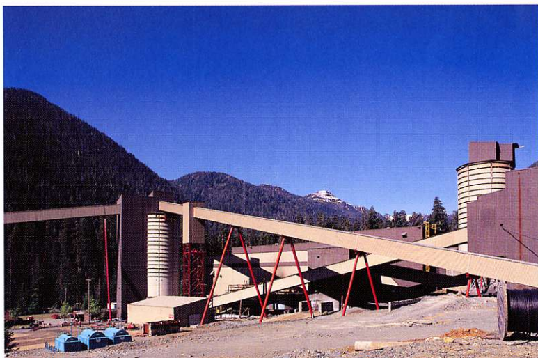
Conveyors transporting ore to mill.
