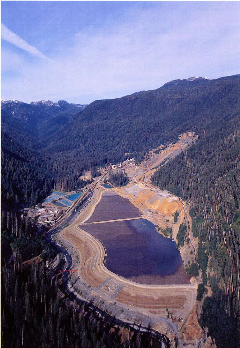
Tailings pond facility.
