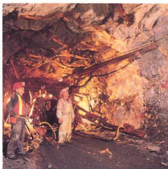
Development progresses on surface and underground
