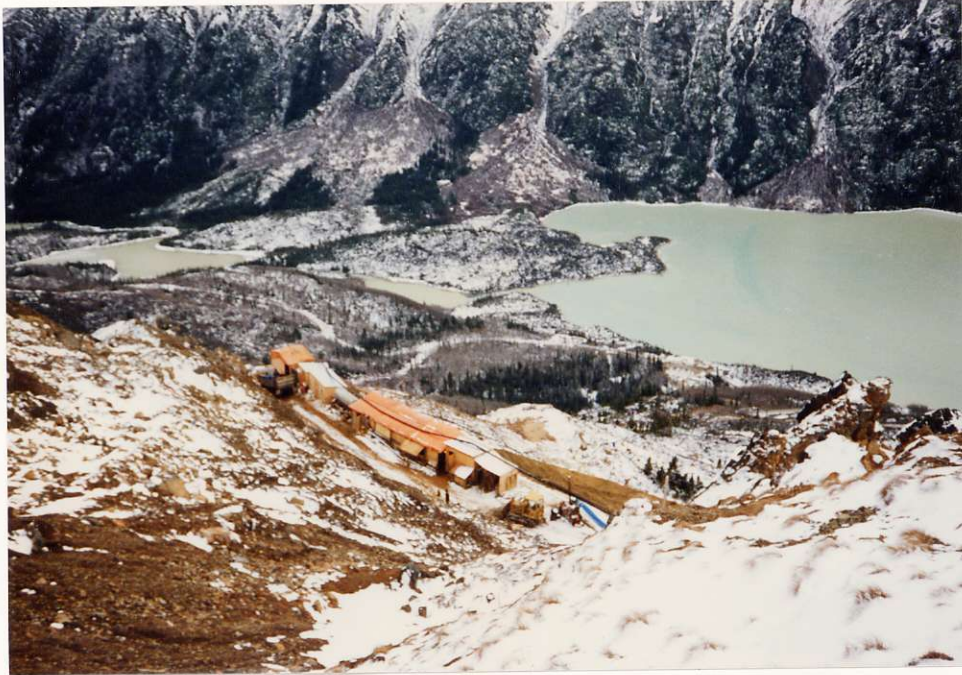
Figure 3. Buildings at portal in the foreground. Blue ventilation pipe leads to portal. Buildings and ground near lake underlain by landslide material. (R#45-13a)
