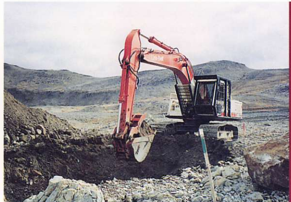
Trenching forms an effective prospecting tool at Golden Bear.
