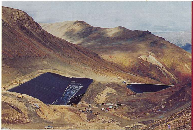
The heap leach pad at Golden Bear was constructed last year.
