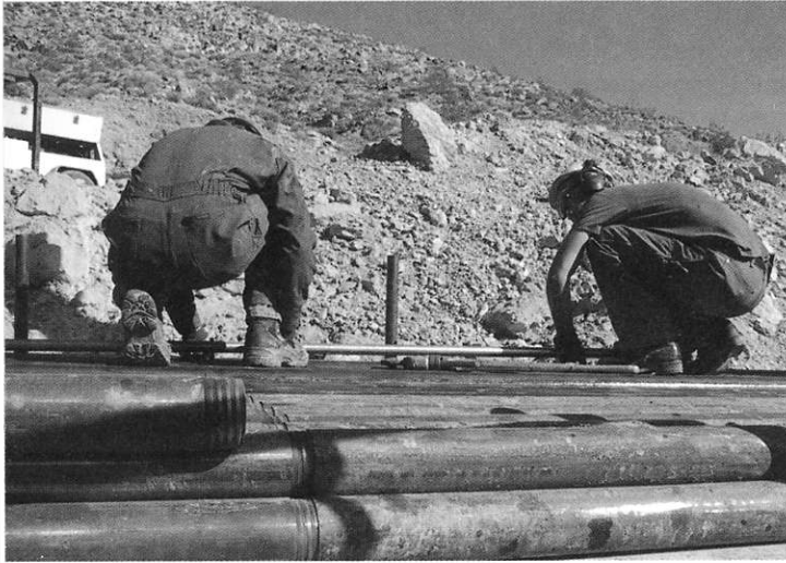
Preparation of diamond drilling equipment
