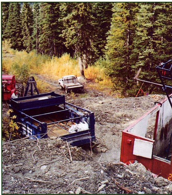
Drilling on Cow Mountain
