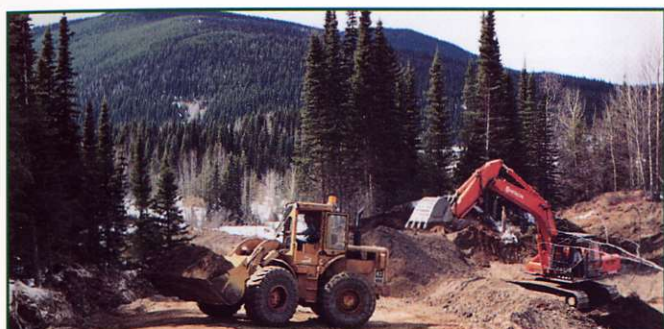
Road building on Cow Mountain with Island Mountain in the background
