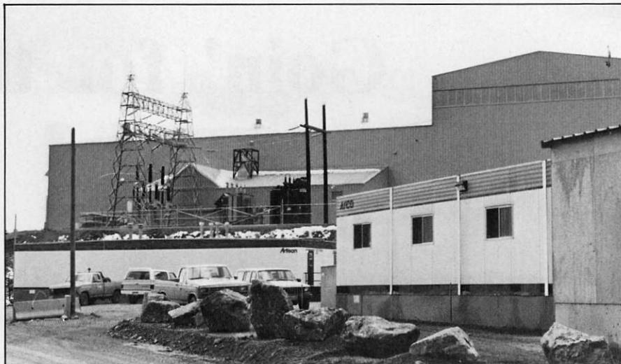
The main mill building at Nickel Plate. It took Mascot less than a year to develop and construct the mine and mill operation.
