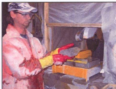
Core cutting is done on site
