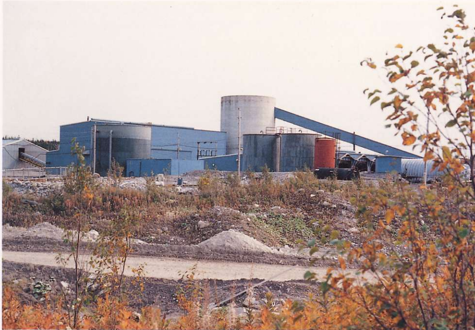
Newfoundland Zinc Mine surface facilities.
