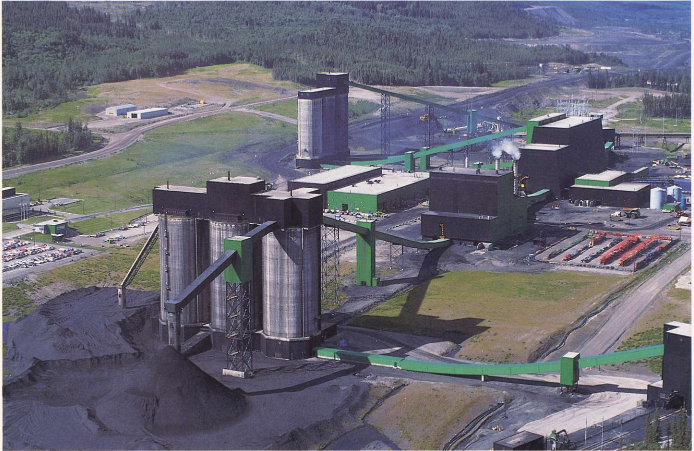
■ Wash plant at the Quintette coal mine, with coal storage silos in foreground.
