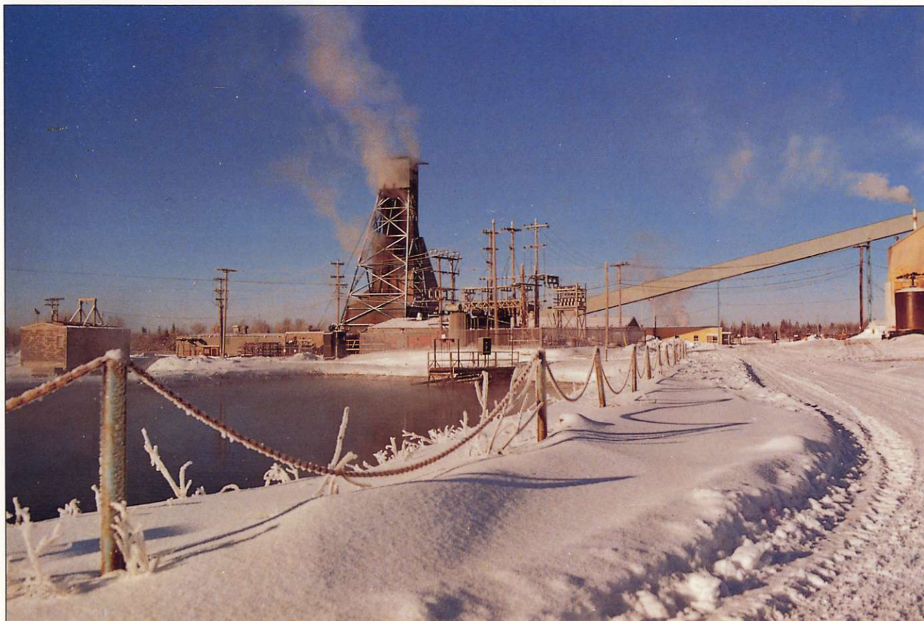
Headframe and shaft house, Niobec niobium mine, Quebec.
