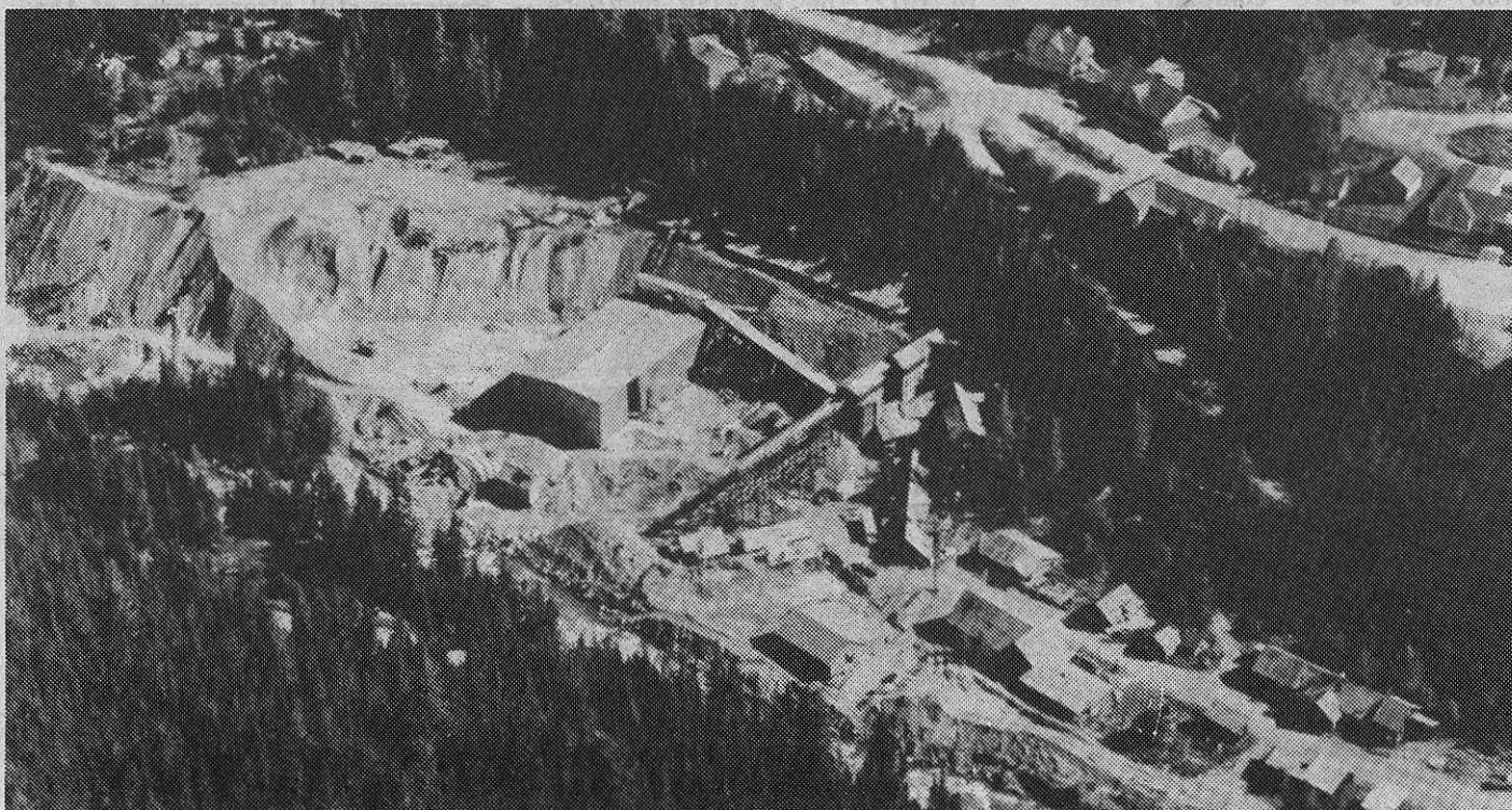
Aerial view of the Bralorne Plant area showing the concentrator building (left), refinery, machine and electrical shops and warehouses. Mine administration buildings are shown in the upper right hand corner.
