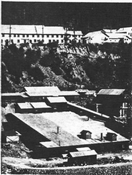
Surface plant, with living accomodation in the background. Bralorne gold mine, Bridge River, B.C.
