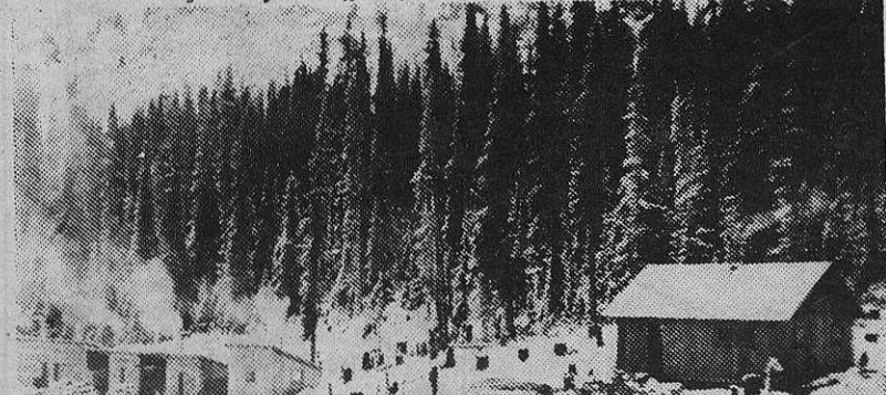
McGILLIVRAY PASS, 1934, [past #26] was site of Standard Mine cabins at 1740 m [5800 ft.] elevation. Then Pioneer Mine was B.C.'s leading lode-gold producer, with 86,622 ounces of gold in 1933 and 89,786 in 1934. Little Gun Lake Lodge was built for Pioneer mine directors in 1934.
