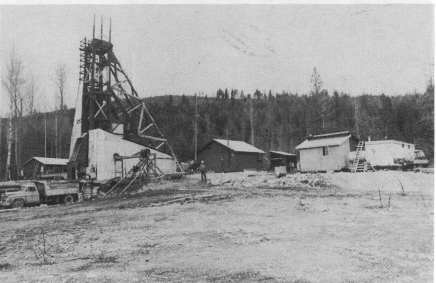
An over-all view of the Jewel property, showing the headframe, hoist house, dry and wash trailer to the right, with the compressor-generator in the left background.
