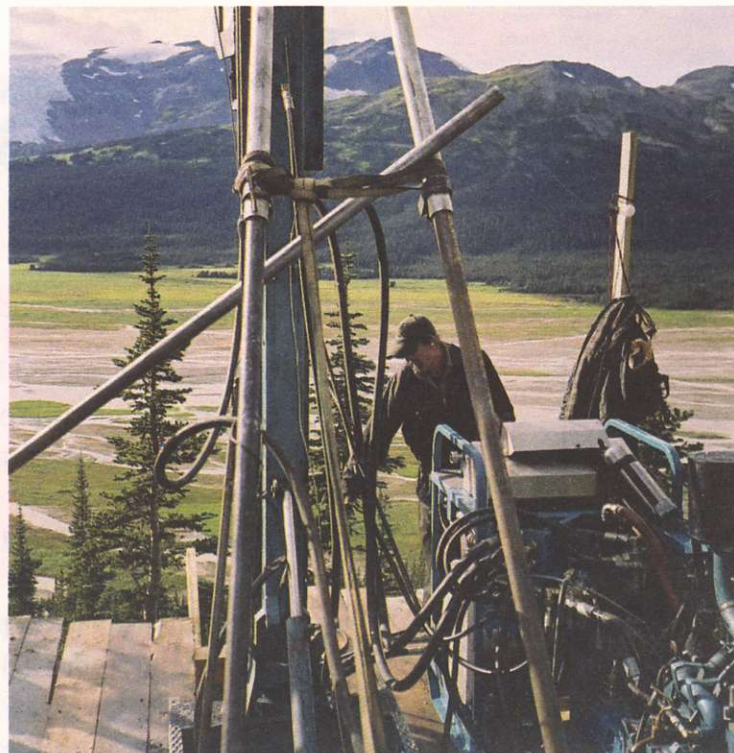
Drill rig on Foremore property in the Eskay/Iskut region of north-western B.C.
