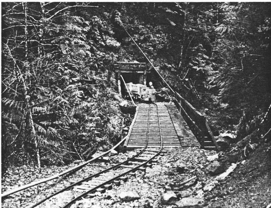
Hauling the high grade ore from the new vein over the new trestle at the 1100 level
