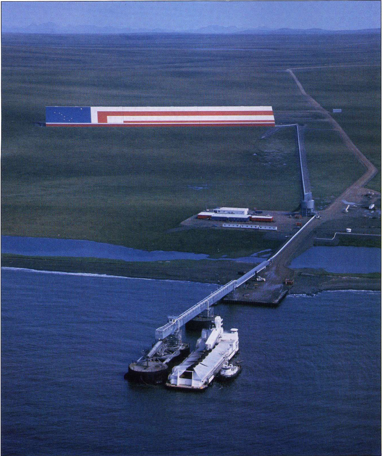
The concentrate storage building dominates the Red Dog port site on the Chukchi Sea. Concentrates are transferred to waiting vessels offshore via specially designed barges.
