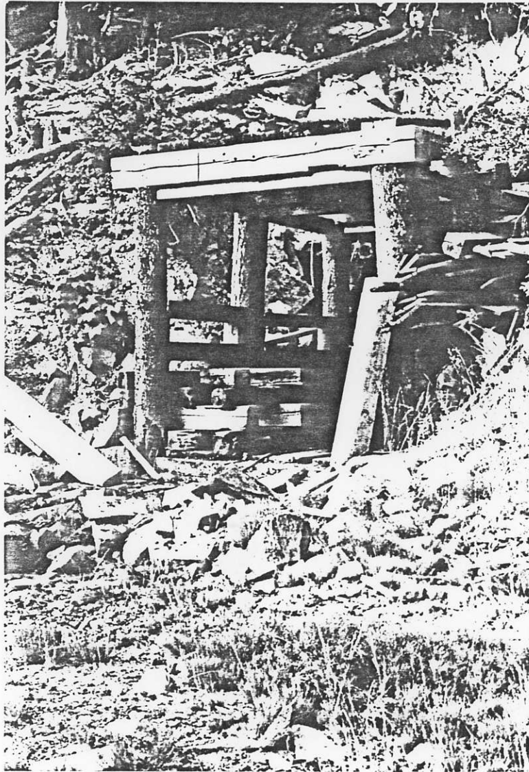
Photo 2. No. 2 adit portal
