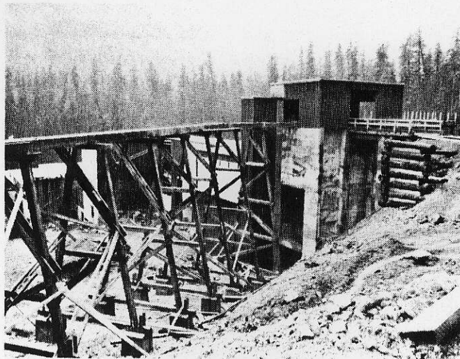
Trestle under construction in 1966 to take ore from Lynx mine portal to the mill, also under construction
