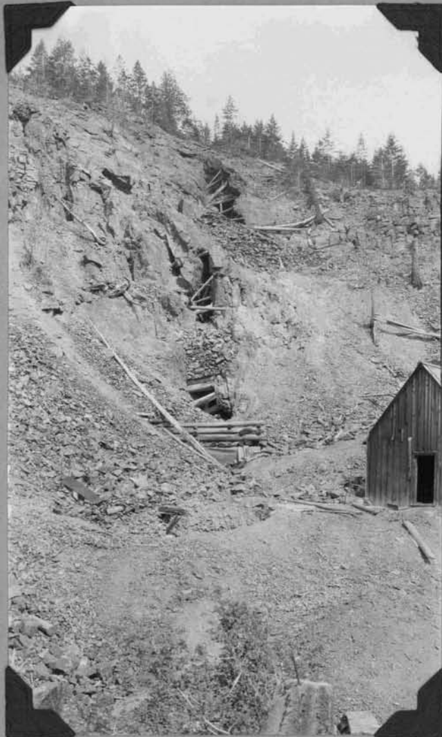
Upper Workings of St. Eugene Mine, showing stopes to surface above #3 Level
