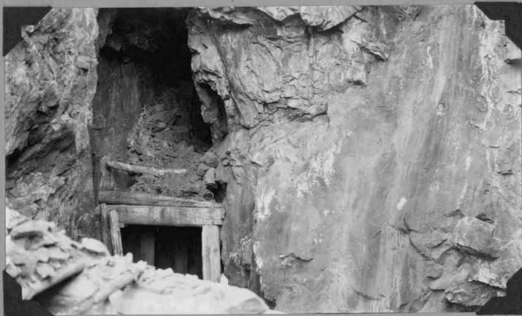
Portal of #8 Adit, St. Eugene Mine, showing big stope along main vein
