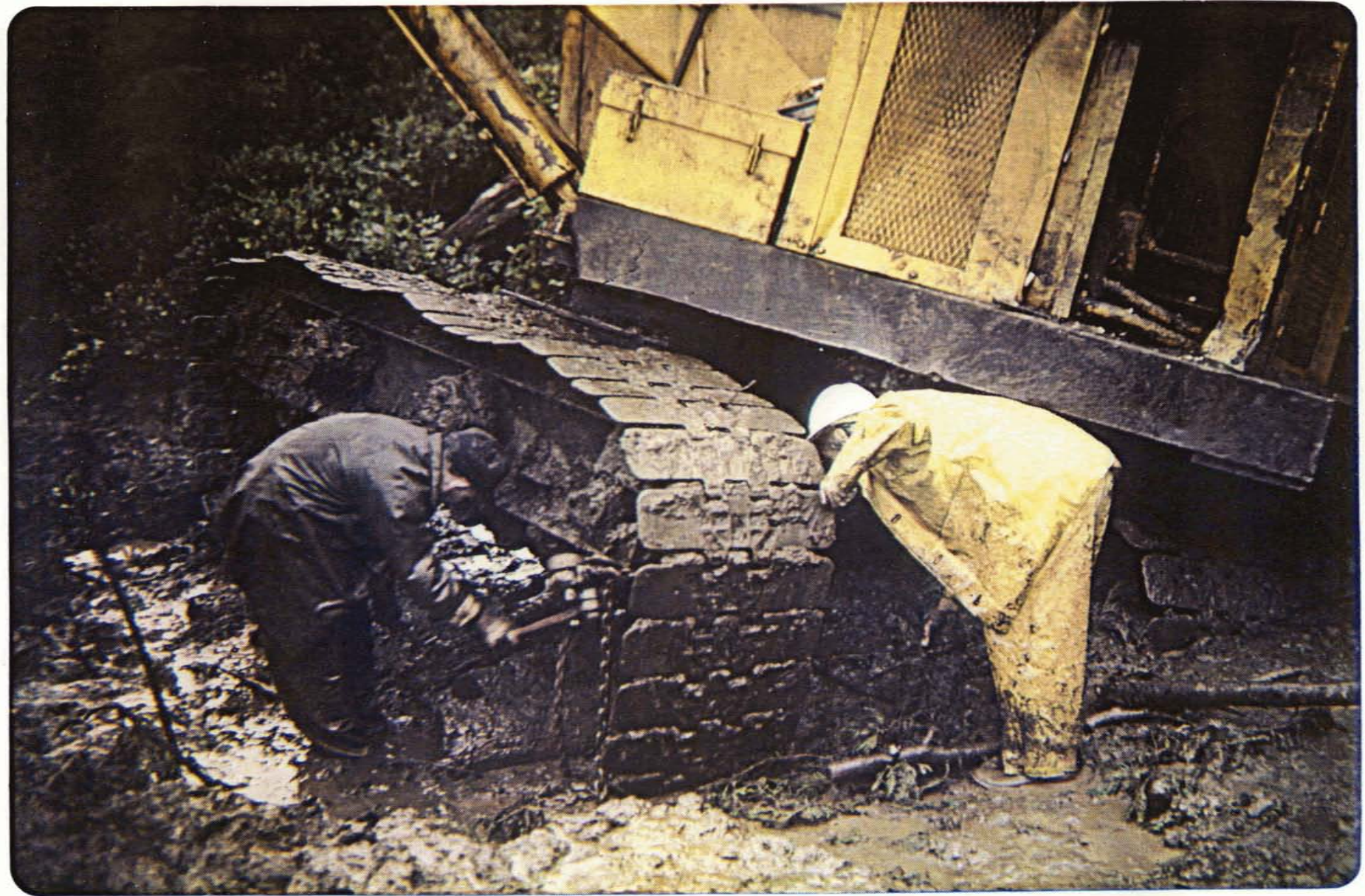
Repairing broken track.
