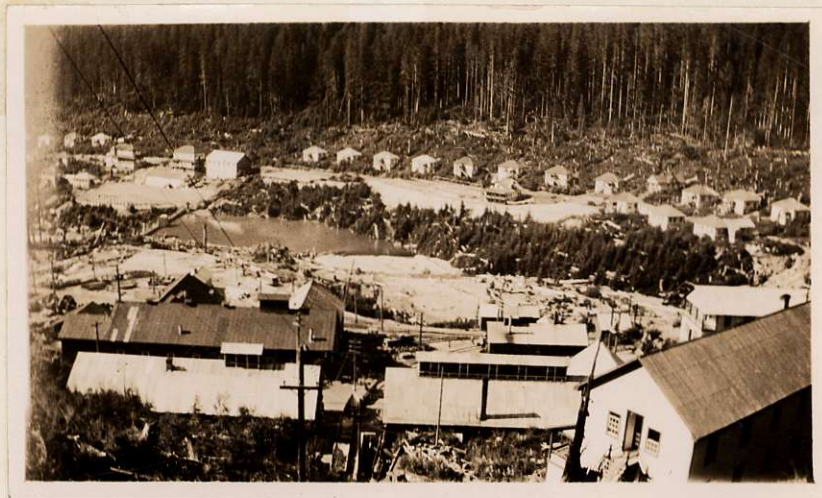
Britannia Townsite taken from above 2200 Portal. 17 ton cars are coming out of mine loaded with ore.
