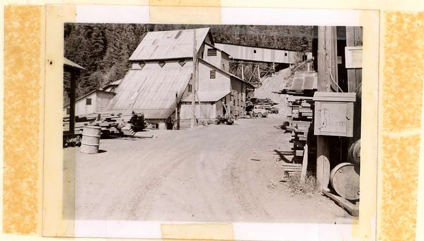
Figure 9. The Cambourne Lead Zinc Concentrating Mill
