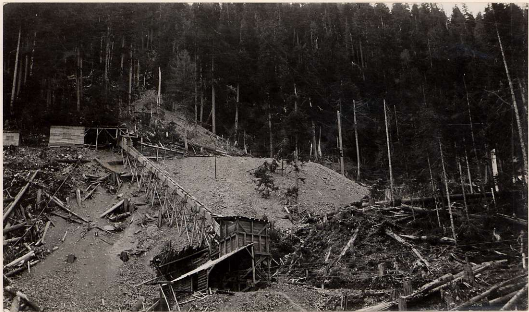
A View of the Main haulage level with the ore shoot & bin in fore ground.
