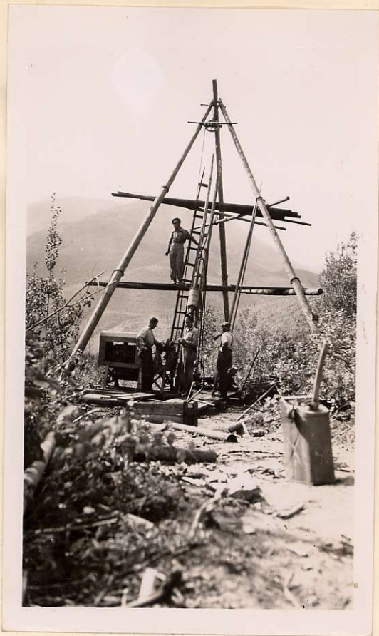
DRIVING PIPE THROUGH OVERBURDEN
