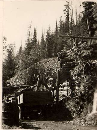
Loading Truck at No. 1 Level Muck Pile and Compressor in background.
