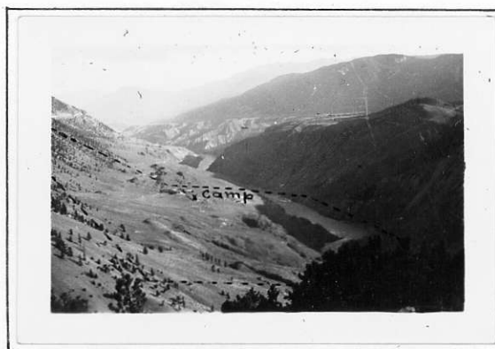
View from railway showing location of property.
