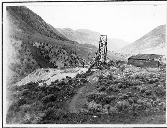
View showing dump, headframe, and compressor shed
