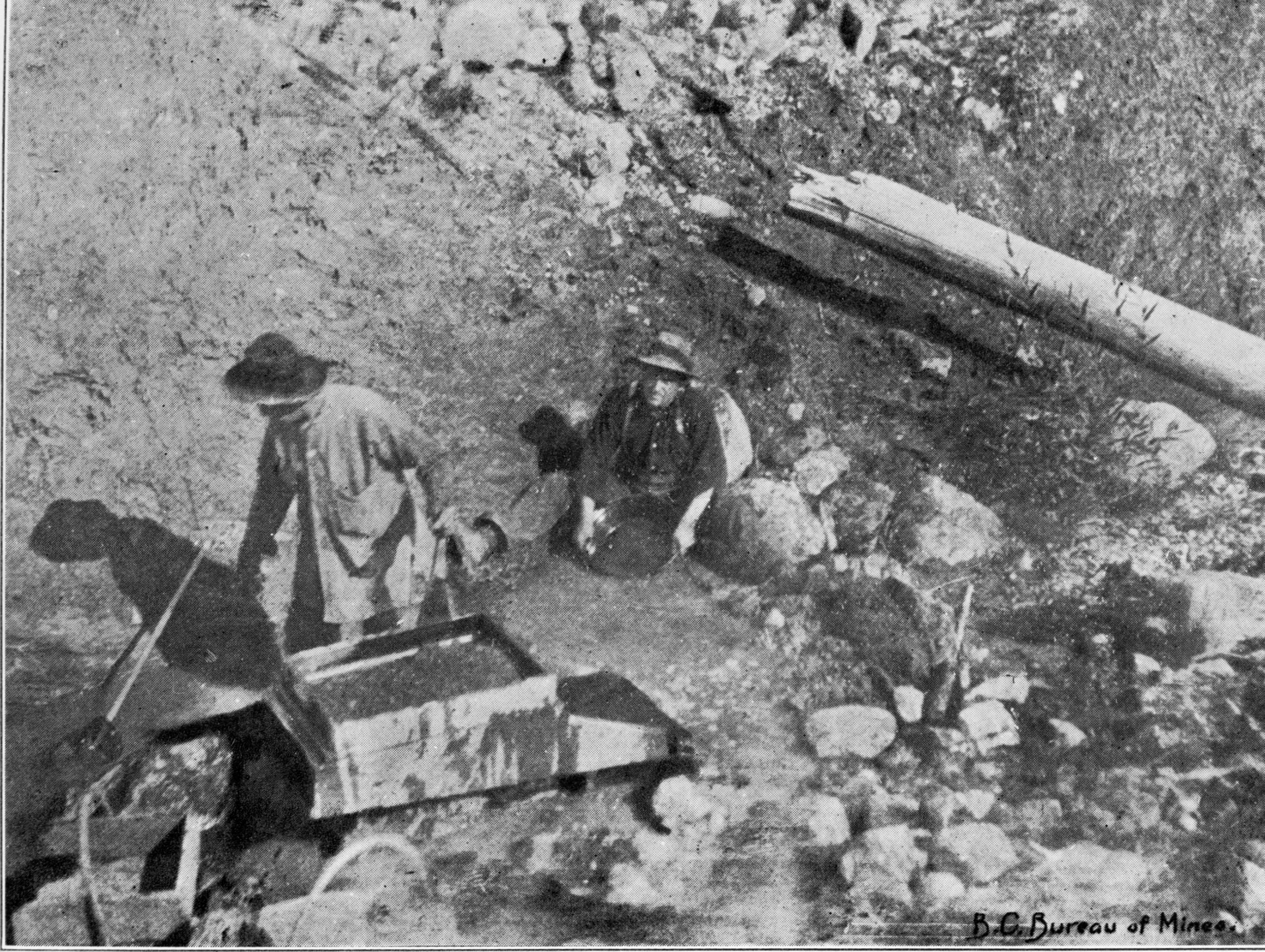
Quesnel Hydraulic Mining Co.—Sampling gravels.
