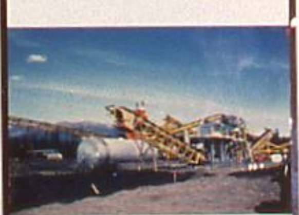
GULF'S COAL-PROCESSING PILOT PLANT NEAR LOST RIDGE
