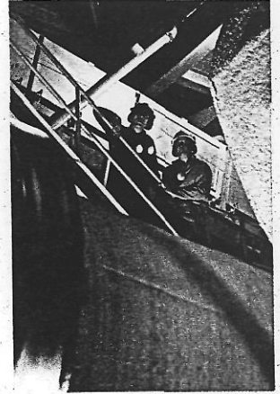
All ore is dried prior to milling, using waste heat from the diesel power plant.
