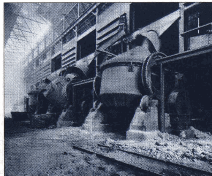
Converters at the Granby smelter, used to make blister copper.
