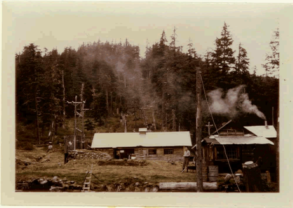
2000 HP hydro-electric plant with operator's house and transformer housing.
