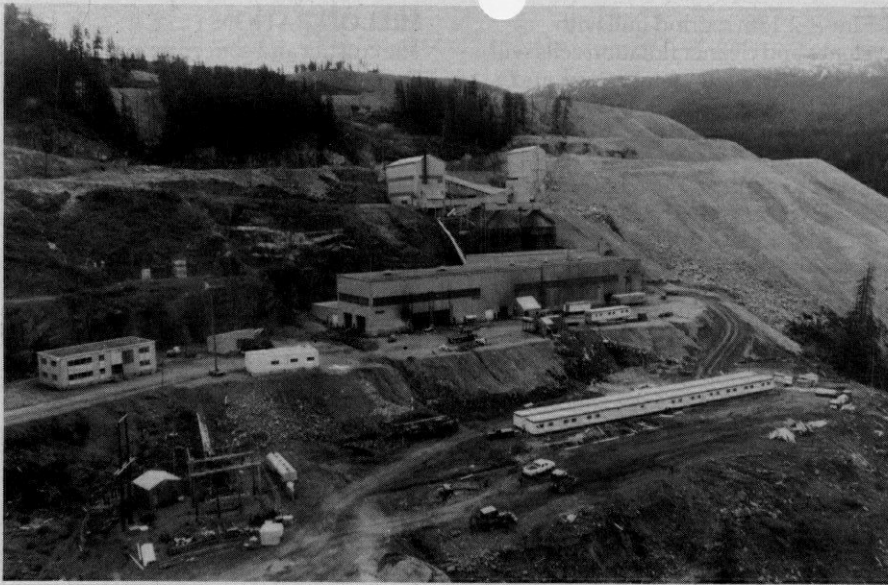
Concentrator building before being expanded and refurbished
