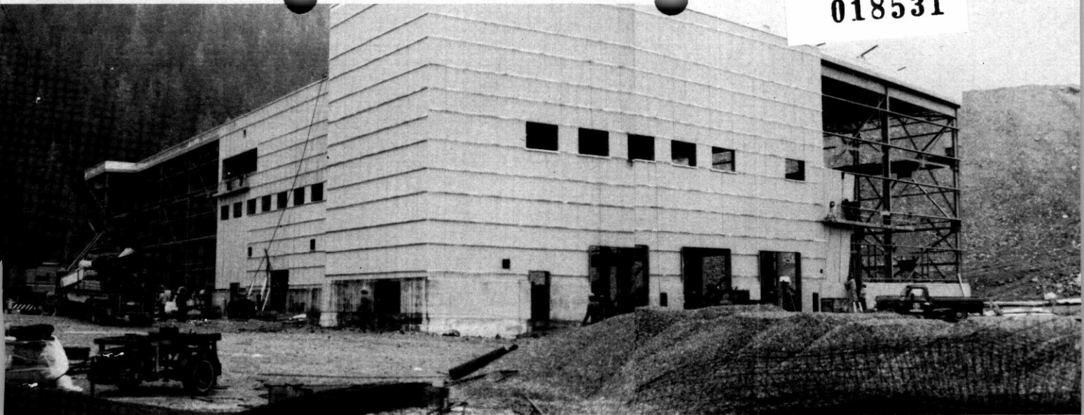
New 35,000 ft 2 mine maintenance complex under construction at Kitsault
