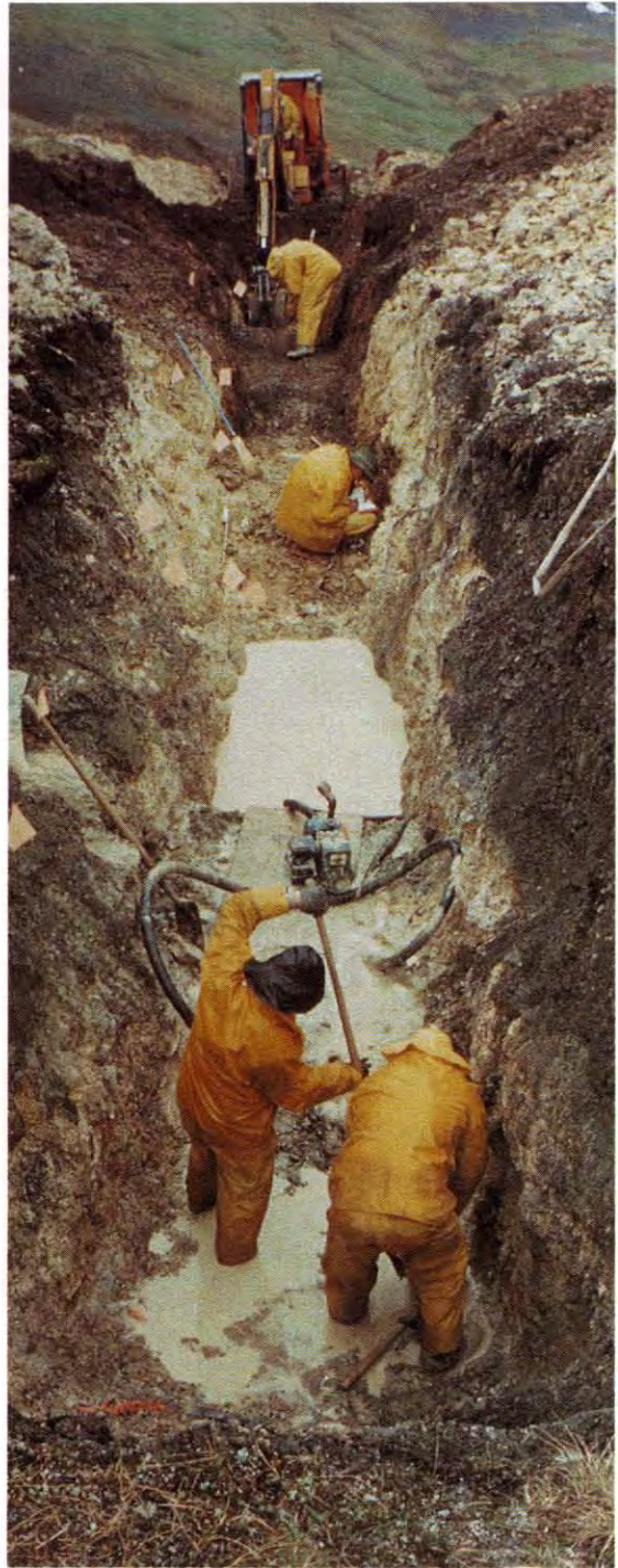
Typical Backhoe Trenching and Surface Sampling
